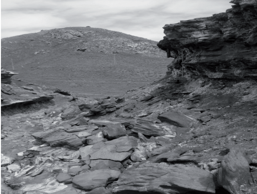
Figure 3: landslide in the flanks of the mining ponds of the studied mining area.
