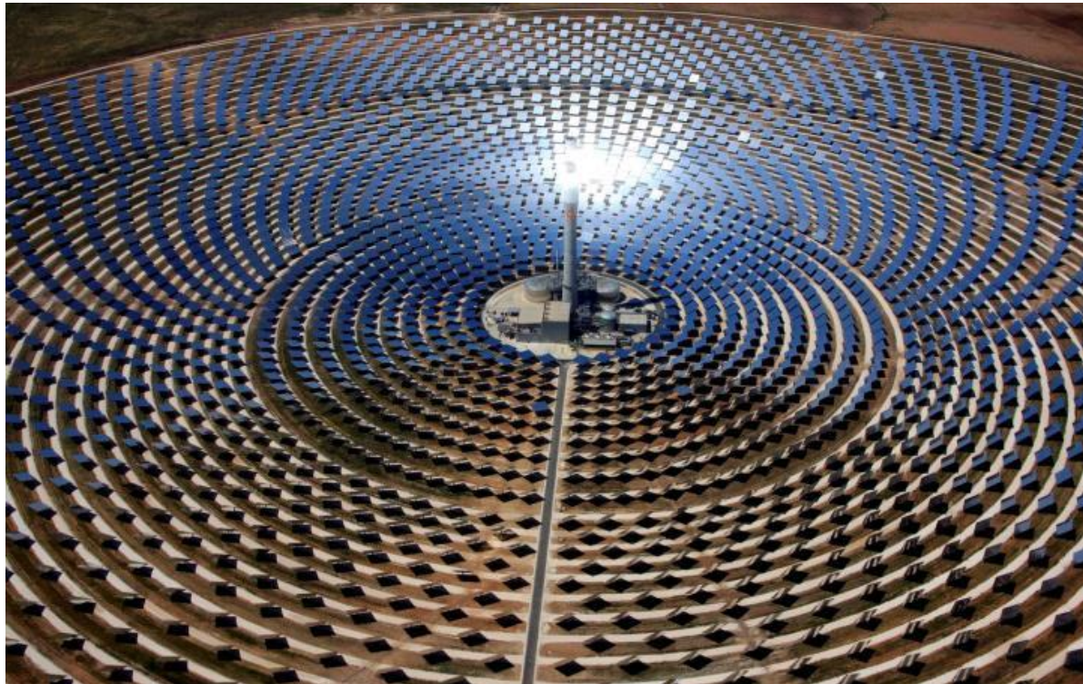
Gemasolar Central Tower CSP plant
