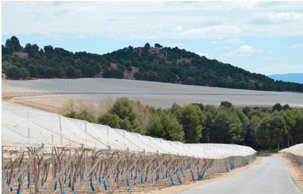
Figure 4. Surface of newly irrigated land (grapes) on the foothills of the Sierra del Gavilán, declared as a Site of Community Interest (LIC) (Archivel, Caravaca de la Cruz). The roads have been conditioned for the entry and exit of heavy load vehicles. Source: Authors.
