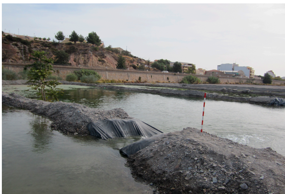
Figure 5. Cultural practices with the construction of ponds in the Rambla of Nogalte favor infiltration and increase the sub-surface flow extracted by the Caño-Contracaño System. Source: Authors (3 November 2022).
