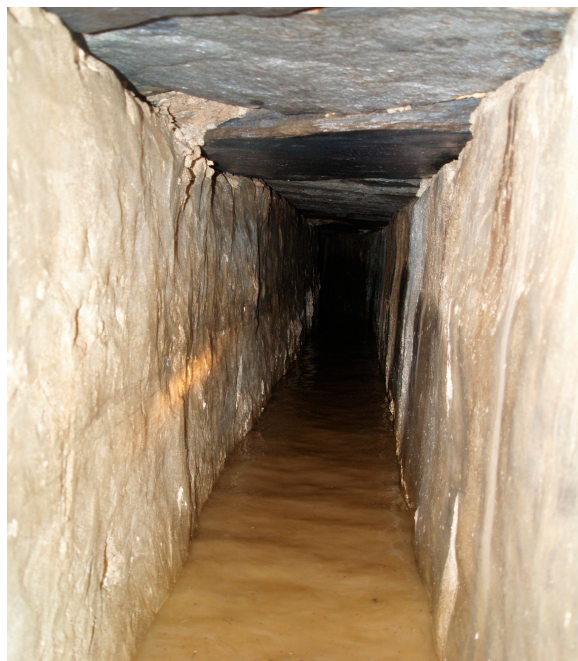
Figure 3. Interior of the Contracaño gallery (Puerto Lumbreras). Source: Authors (2 April 2004).
