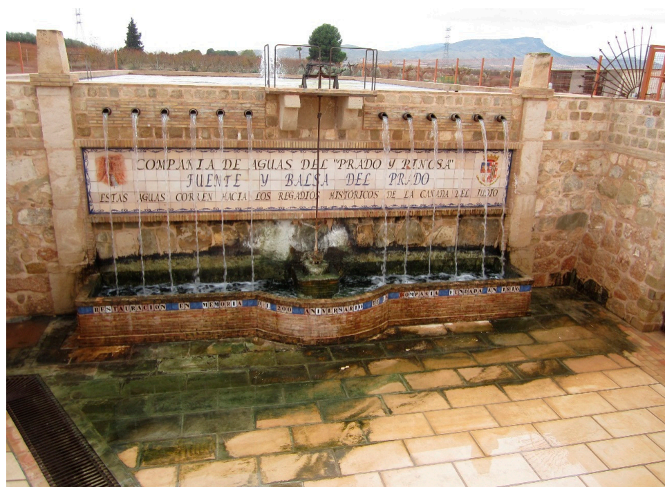
Figure 4. Restoration of the fountain, spouts, pond, and trough of the Compañía de Aguas del Prado y La Pinosa, supplied by the water collected by several mines with mirrors in Jumilla (Region of Murcia). Source: Authors (2 December 2022).
