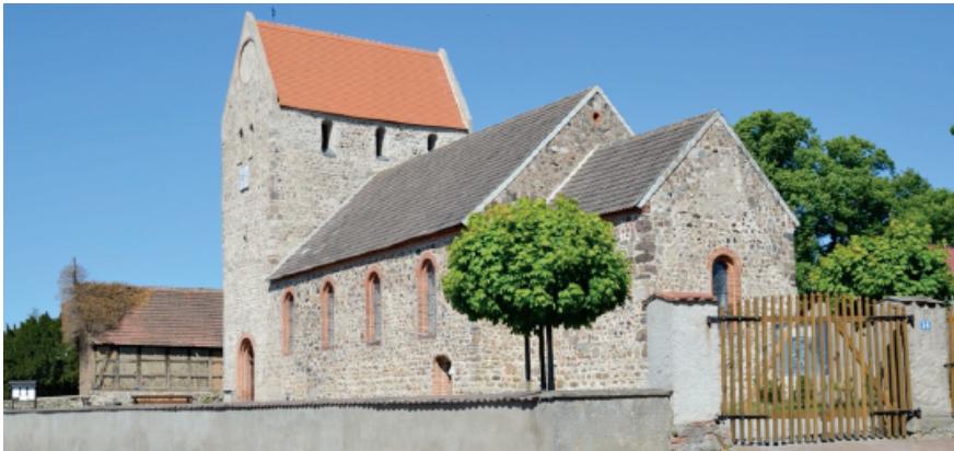
Fig. 5. Church constructed by field stone in Altensalzwedel, Altmark region (photo: Hansjörg Küster).
