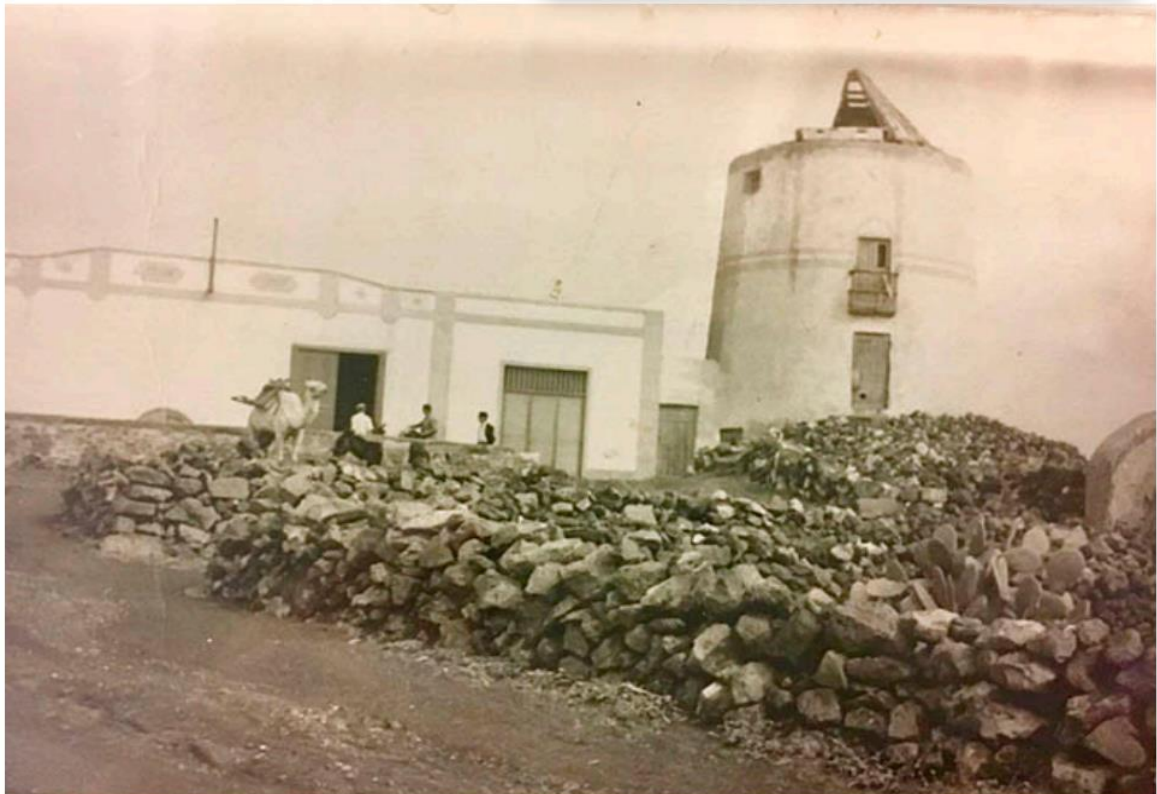
Figure 3.14. Flour mill of SB (1870), erected by Baltasar Fermín and acquired by José María Gil in 1919, today declared a Site of Cultural Interest (BIC)
