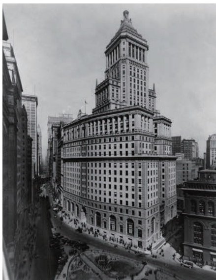
Figura 23. Standard Oil Building de Nueva York.
